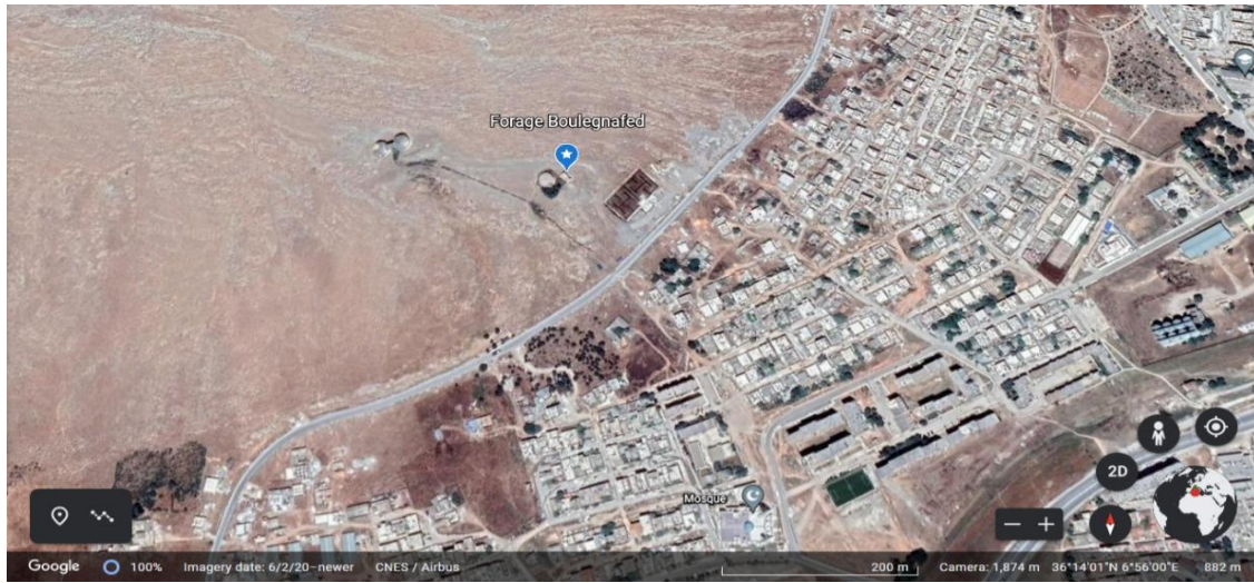
Figure 8. Image satellitaire de la station pompage Boulegnafed (Google Earth, 2021).
